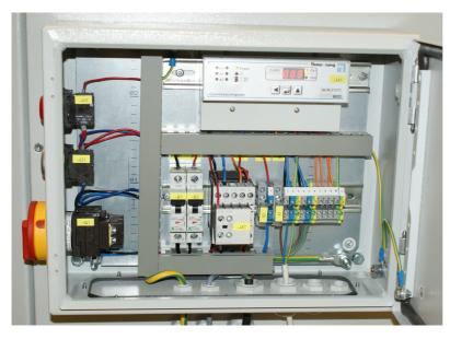
The **LCS1** is used for monitoring the interior of cabinets which contain gas-carrying components such as those existing in gas analyzing systems for mine gas, waste landfill site gas, digester gas or biogas.
